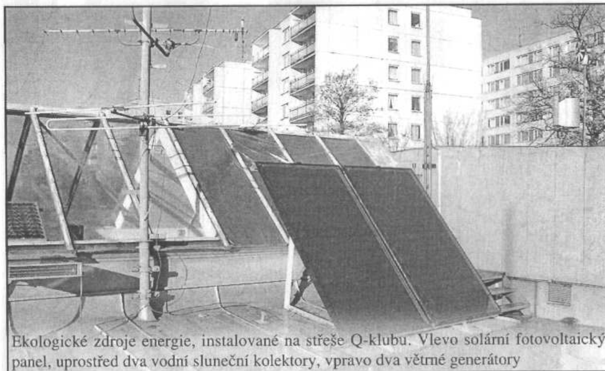
Ecological power sources on the roof, left: solar battery panels, centre: two sun water heating panels, right: two wind generators
